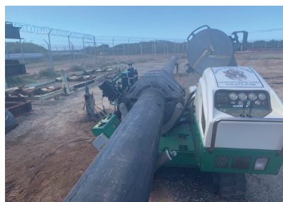
HDPE Fusion Equipment and Training
