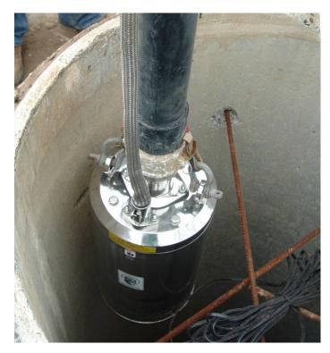
Mody Pumps produce a pump that is specifically designed for this purpose (model # G506T/316SS, 4" Stainless, up to 125gpm or up to 170' of head). This pump has been sold to landfills across the country but this is the first one to enter the Hawaiian Islands.
