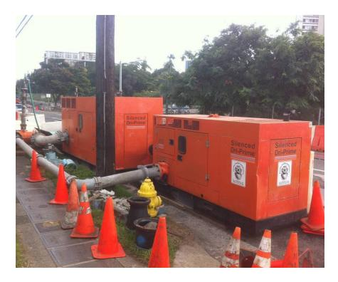
The wastewater sewer system on School St. picks up sewer flows from most of Liliha. This line is capable of flows up to 17.3 million gallons per day plus lateral lines totaling in another 7.2 million gallons per day. This project was set-up using (3) 12" Electric DPC300 Godwin Dri-Prime pumps, (2) 12" DPC300 Critically Silenced Diesel Godwin Dri-Prime pumps, an 8" CD225M Critically Silenced Diesel Godwin Dri-Prime and (2) 6" CD150M Godwin diesel Dri-Prime pumps.
