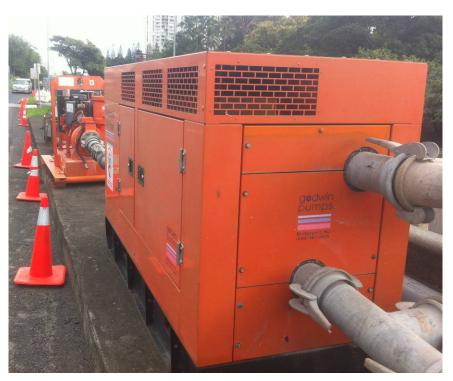
Mira Image Construction used an assortment of Pacific Pump and Power's pre-manufactured manifolds with ARI, air relief vents, 18" HDPE discharge piping and pneumatic pipe plugs. In addition, PPP expertise was provided to assist in planning and setting up a very successful bypass.
