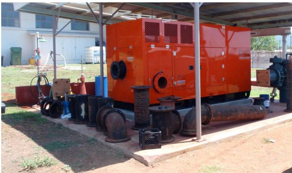
12" x 12" CD300M Critically Silenced Pump, Skid Mounted
