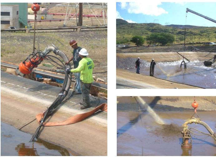
With the remotely controlled Slurry Gate Pump, BSE operators loosened up years of sludge, and blended it into manageable slurry. It was then pumped approximately
