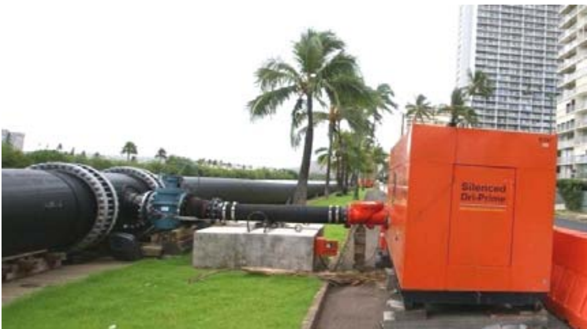
Bottom Left : Hawaiian Dredging – Ala Wai Canal Bypass Seven 12" DPC300 Critically Silenced Pumps
