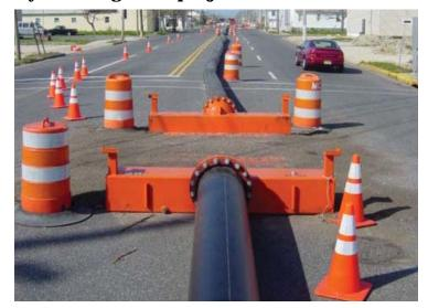
Godwin road ramps are designed to provide easy crossing of a pipeline in lowtraffic areas and can be used in a series to re-route traffic patterns.
