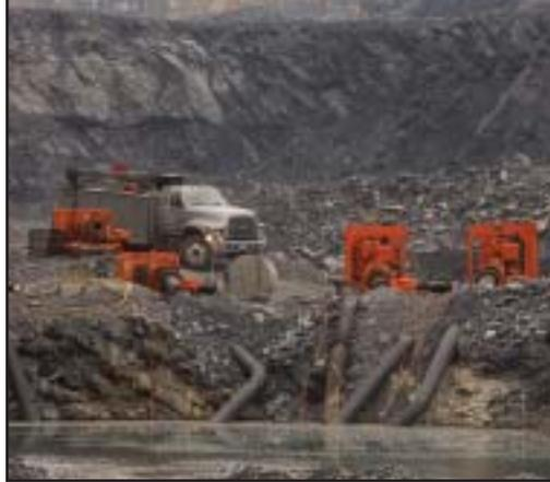
30,000 gallons per minute coming from the F Level and bypassing the flow around the current East Dam retention lake and removing 100 million gallons of water from a portion of the East Dam retention lake so that a dam-like wall could be built to retain a smaller East Dam retention pond.
