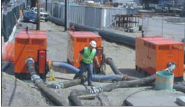
Boston's Bremen Street pump station housed three of 23 Godwin Critically Silenced Dri-Prime pumps. Pumps at six pump stations worked to handle 32 mgd of combined sewer overflow. The project marked the largest sound-attenuated pumping system installed in the United States.
