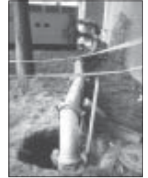
CD150M 6" (150mm) Dri-Prime for Stormwater Sewer Bypass
